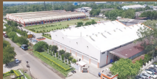
PIX Transmissions Limited Wrapped Belt Plant
